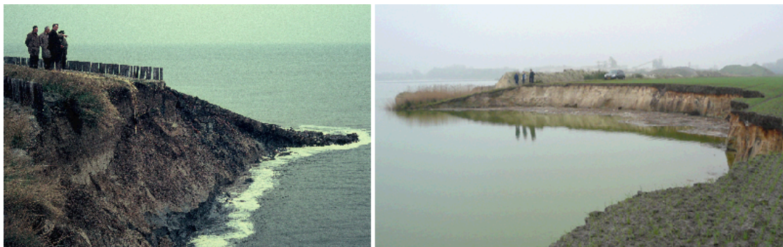
Figure 1.1: Examples of damage to a dike due to a flow slide
