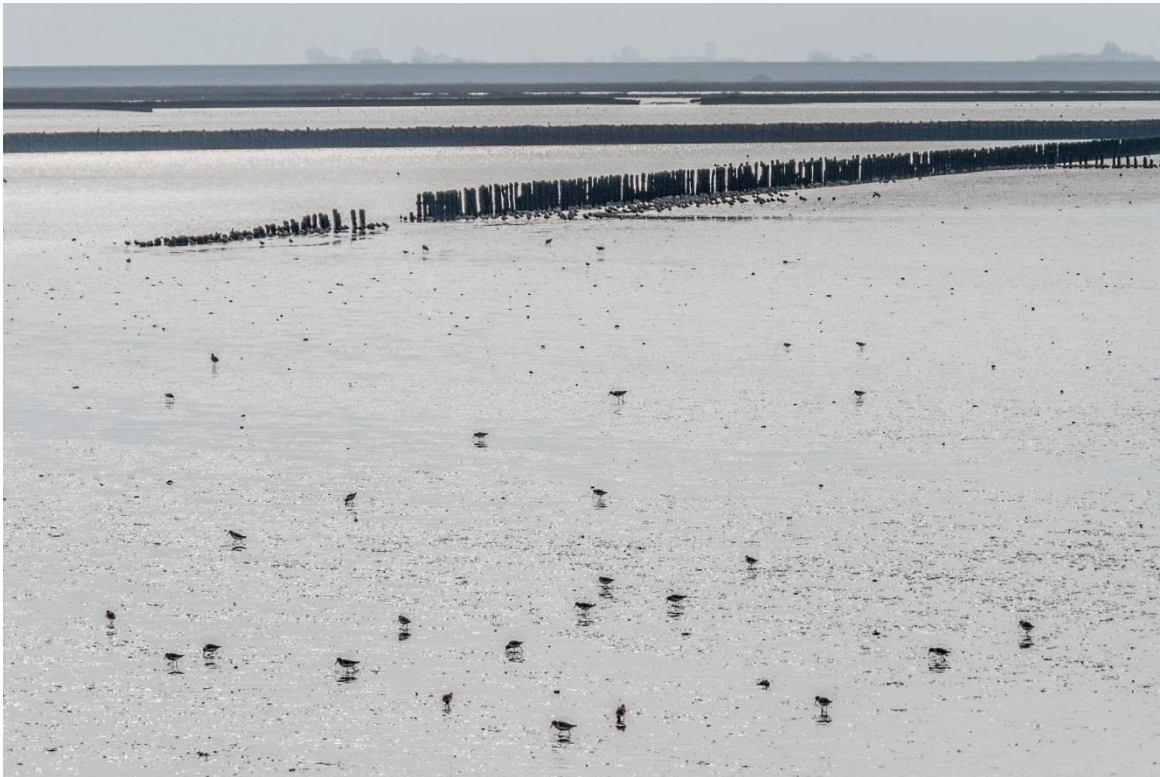
Figure A.4 Holwerd, near the mainland: brushwood groins, 8-10-2014. (RWS, Harry van Reeken)
